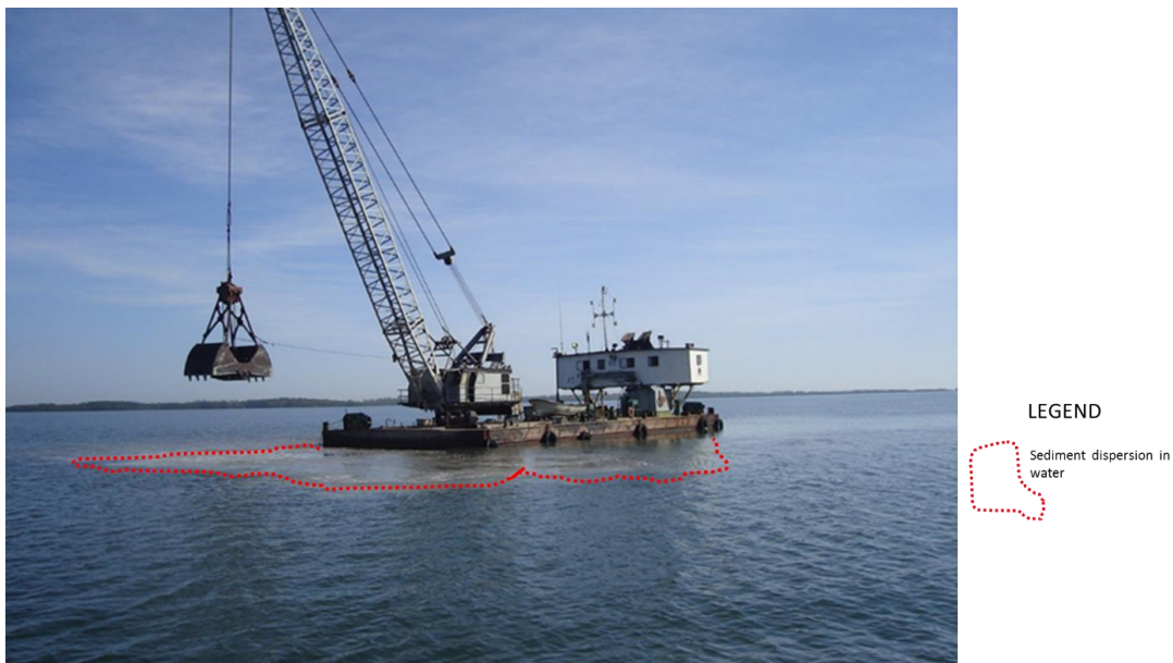
Figure 2. Excavator used for dredging carbonated silts.
