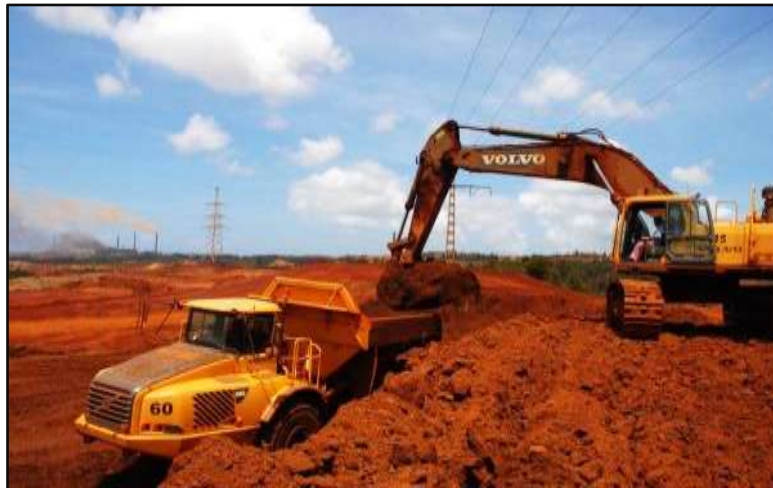
Figure 3. Open-pit exploitation system. Source: Fonseca-Aguilar (2024).
