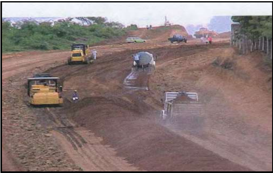
Figure 5. Construction of the base grounds. Source: Fonseca-Aguilar (2024).
