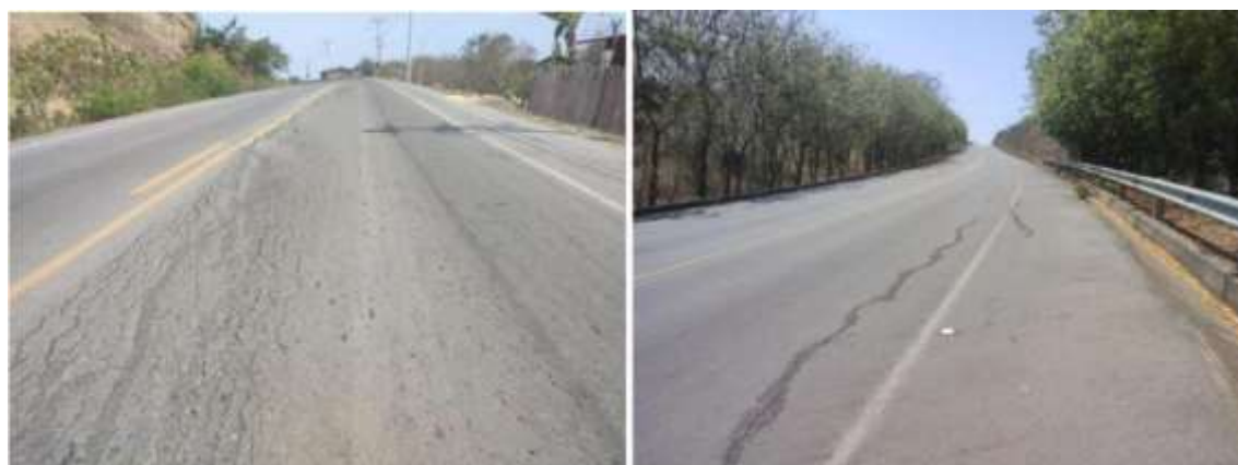
Figure 2. Detected cracks on the road based in visual inspection (Source: own elaboration).
